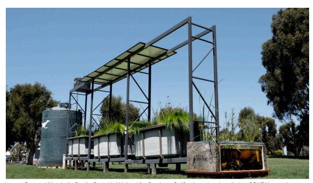
Lauren Bon and Metabolic Studio *Portable Wetland for Southern California* system installed at CSUDH uses three "cells" filled with scoria and native wetland plants native that will filter and treat water from the university's water supply.
